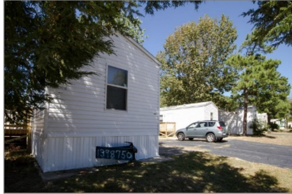
One of several MHUs provided by FEMA in Crestwood, New Jersey following Hurricane Sandy.
