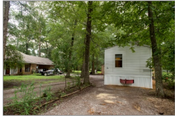
MHU sits next to a residence in Zachary, Louisiana after flooding
