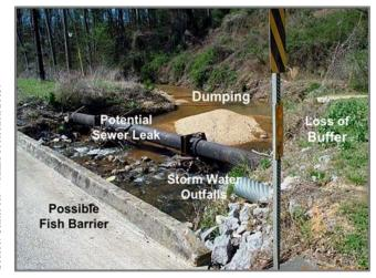
Figure 3-14. Potential Sources of Stream Degradation
