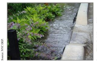
Photo A4-3. Bioswale During a Storm Event
