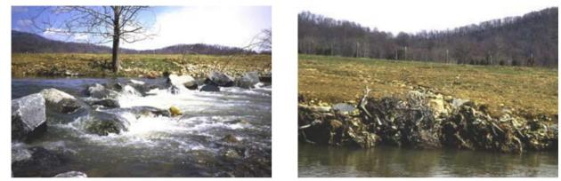
Photo 3-11. (L) Weir Constructed on the Channel; (R) Rootwads in the Channel Rose River, Madison County, VA
