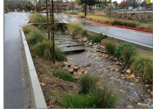
Photo 3-15. Example of Stormwater Storage during a Rainfall
